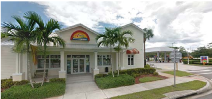
Figure Sec. 90-36.13 Service station examples of pumps to the side of the building
